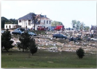
Concrete Home After Tornado
